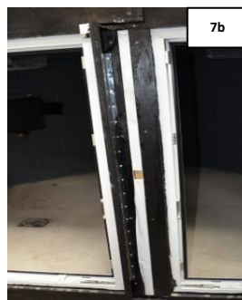
Figure 7a-7c: Showing a very simple way of managing a venomous species off show, by dividing the entire enclosure. The board slides in to place, shutting off and isolating the animal in another part of the enclosure.
